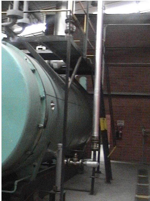
FIGURA 1.2 CALDERO PIROTUBULAR DE 600 BHP.
