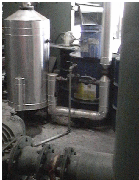
FIGURA 1.16 TANQUE FLASH SINGLE FABER C
