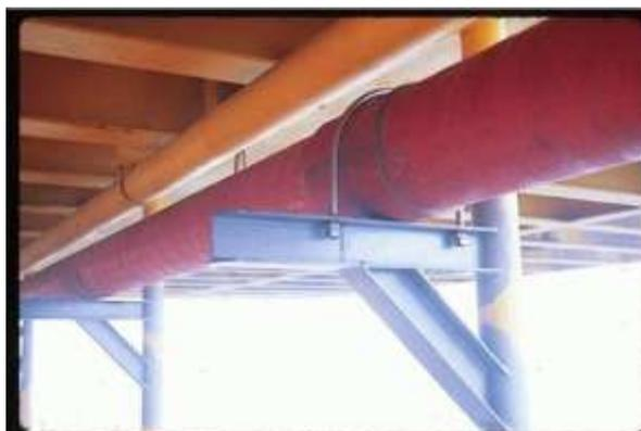
**FIGURA 6.1 SOPORTE TUBERÍA SISTEMA CONTRA INCENDIO**
