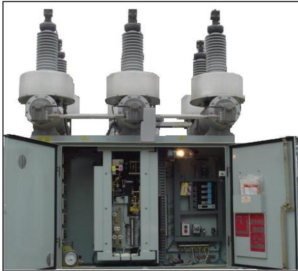
**Fig. 4.15 Interruptor en gas SF6 (GCB)**
