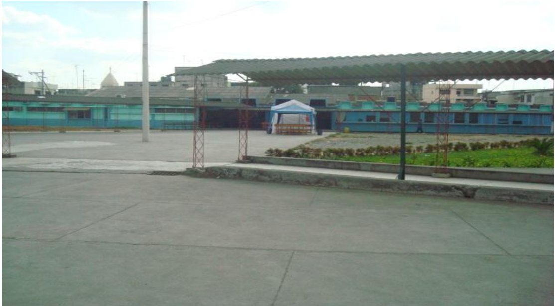
Figura A.1-2 Patio central del hospital
