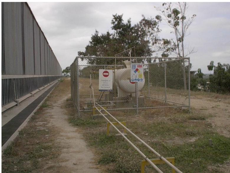
**FIGURA 2.4: TANQUE DE GLP (SALA DE ADITIVOS)**
