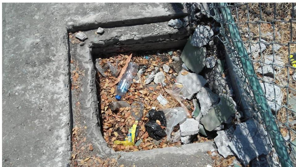
**Figura 5.65 Caja RSC1 Colapsada.**
