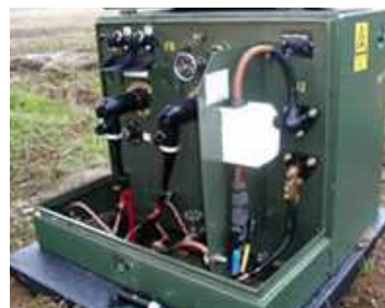
Figura 8. Transformador Pad-Mounted instalado
