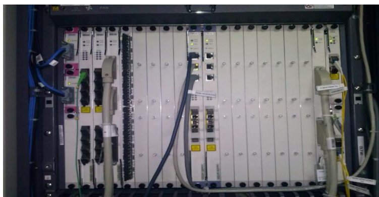
Figura 4.30: OLT Huawei MA5600T.
