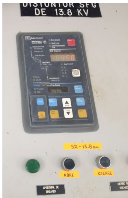
Fig 1.8 Relé Cutler Hammer Digitrip 3000
