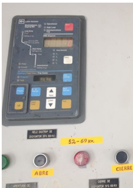
Fig. 1.7 Relé Cutler Hammer Digitrip MV
