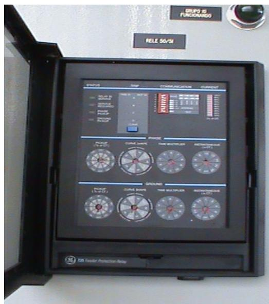
Figura 1.8. General Electric 735 Feeder Protection
