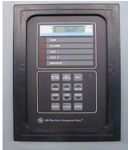
Figura 1.7. MOTOR MANAGEMENT RELAY 269
