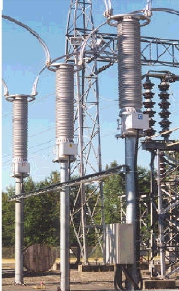
*TRANSDUCTOR OPTICO DE VOLTAJE Y CORRIENTE
