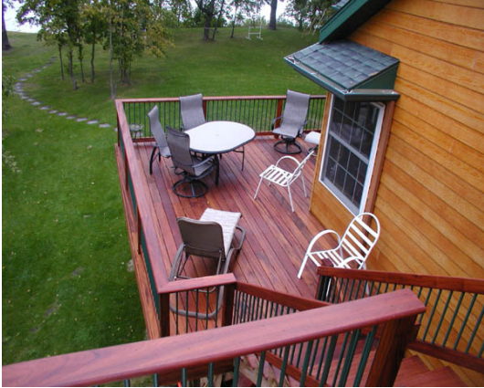
Foto No. 12: Decking de Calvellin- TigerWood ( Astronium Graveolens )
