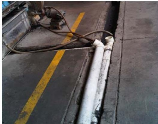
**FIGURA 4.12 TUBERÍAS DESORDENADAS**
