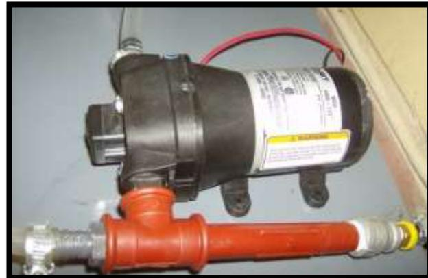
**Figura 4.3 – Bomba y bypass**
