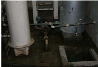
**FIGURA 3.15 BOMBA CISTERNA TORRE DE ENFRIAMIENTO**
