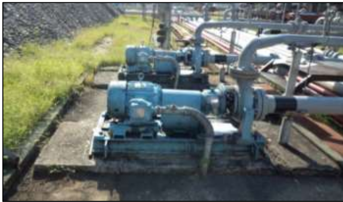
FIGURA 2.10: Bomba Booster
