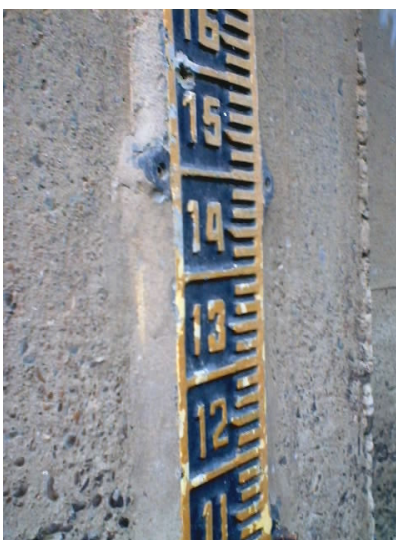
Photo 3.1. Level marker attached to a bridge's pile
