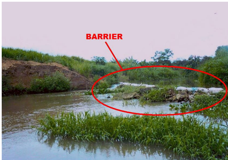
Photo 3.3. Barrier built by a banana farmer to protect a pump uptake
