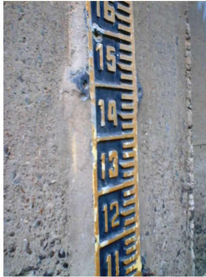
Photo 3.1. Level marker attached to a bridge's pile
