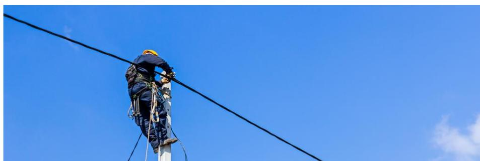
**Figura 4.6: Cable aéreo ADSS [53]**
