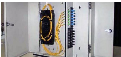
Figura 3.19 Caja Terminal NAP de exterior [34]
