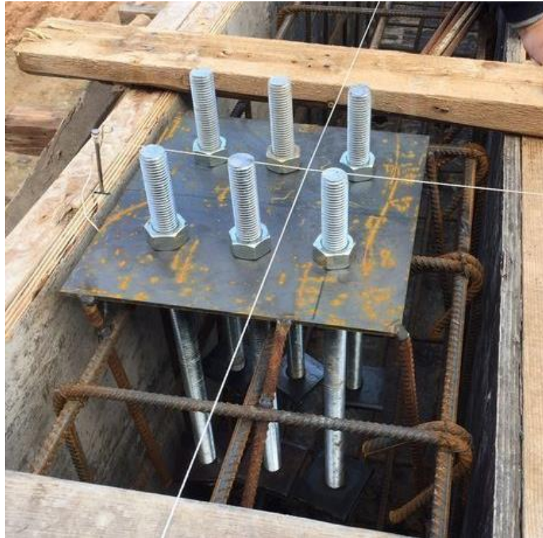
Figura 3.64 Placa de anclaje columna-viga IPE [Engineering Discoveries, 2020]
