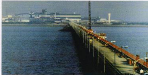
Fig. 4: Straight portion of pipe conveyor at jetty
