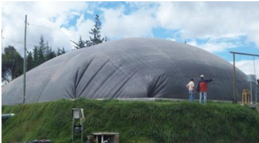
Figura 2 Biodigestor San Francisco, Latacunga-Ecuador
