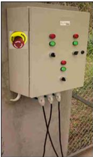
Figura 1. Panel de Control
