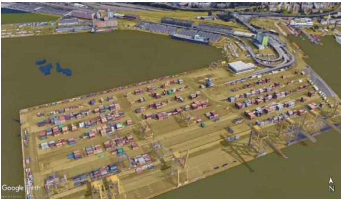
Figure 3.24 Flooding of Trieste Commercial Port. (Author`s, 2020)
